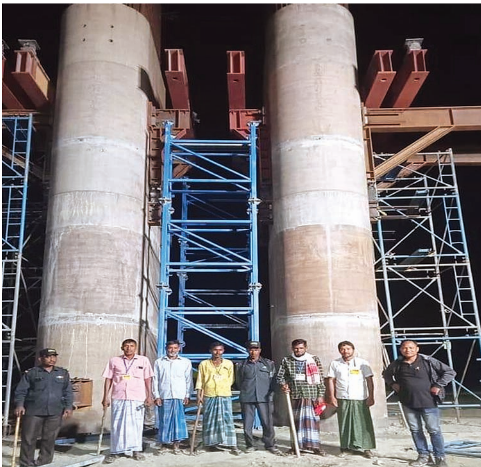
Guarding construction site of Phulbari Bridge by VDP volunteers in Dhubri District.
